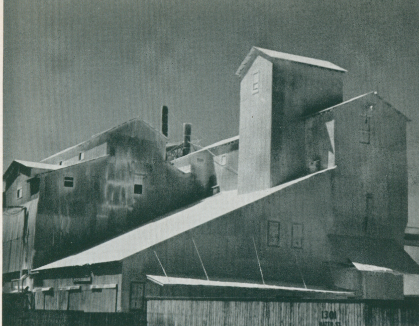
Old Lime Mill
