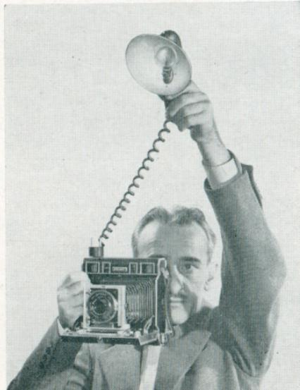
*The "Coilflash" FLASH Reflector Unit enables the photographer to obtain desirable lighting results on portraits and other close-up subjects. The coiled wire in the wire chamber (handle) will stretch to over 36 inches—more than arm's length for the average man. It disappears into the chamber when reflector is returned to its base.*
