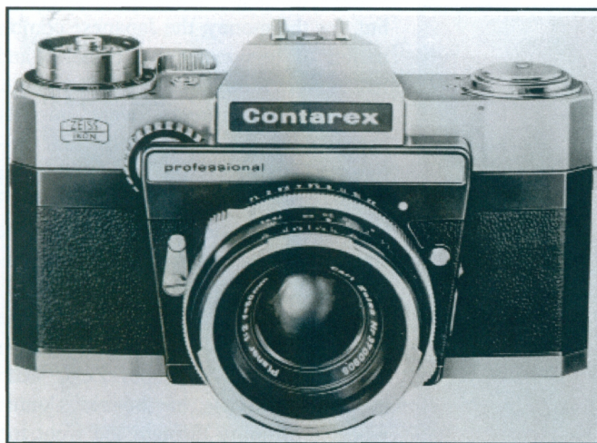
The Contarex Professional (above) and the Contarex Super (right). The Professional is shown with the 50 mm f/2 Blitz Planar, which has built-in flash synchronization. Figure 6
