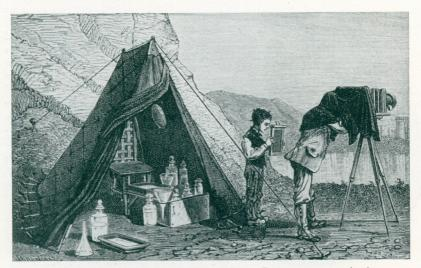
Before the Kodak and film photography were born. Equipment necessary for the amateur during the "wet plate" days
