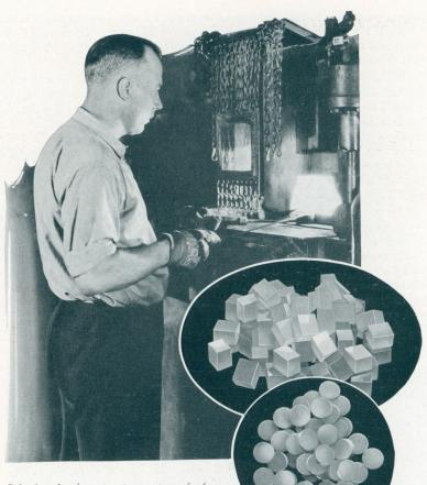
Softening the glass at a temperature of 1600 degrees so that it can be molded and pressed into discs. Oval shows the way the glass looks before being placed in the furnace, and circle the molded and pressed discs
