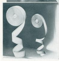
Cutting motion picture film to its proper width of 35 millimeters. Insert shows a finished 250-foot roll of standard film and a 100-foot roll of Ciné-Kodak Safety Film; 4000 pictures are possible on each length
