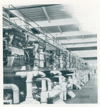
Battery of coating machines which spread the film "dope" on the rims of huge polished wheels to form the transparent film base
