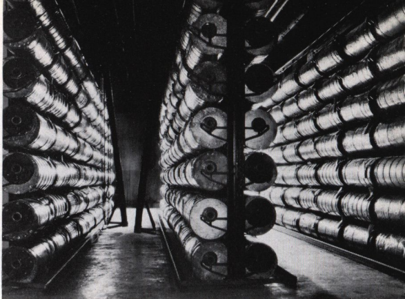
Rolls of film base in storage prior to receiving the sensitive emulsion coating.
