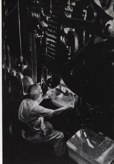
Stamping out the tin containers for motion picture film.
