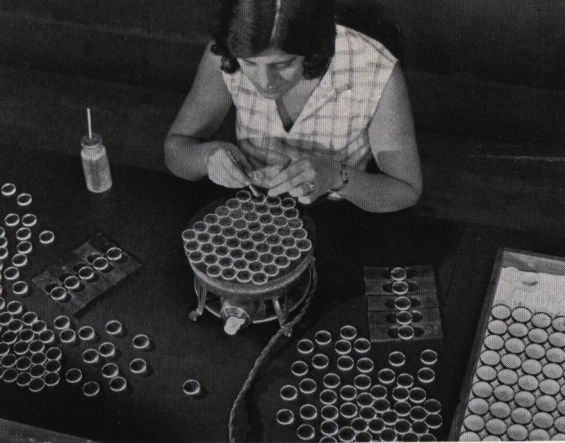
Canada Balsam, softened by heat, is used for cementing together crown and flint glasses. The presence of two kinds of glass in a single lens element corrects certain optical aberrations.
