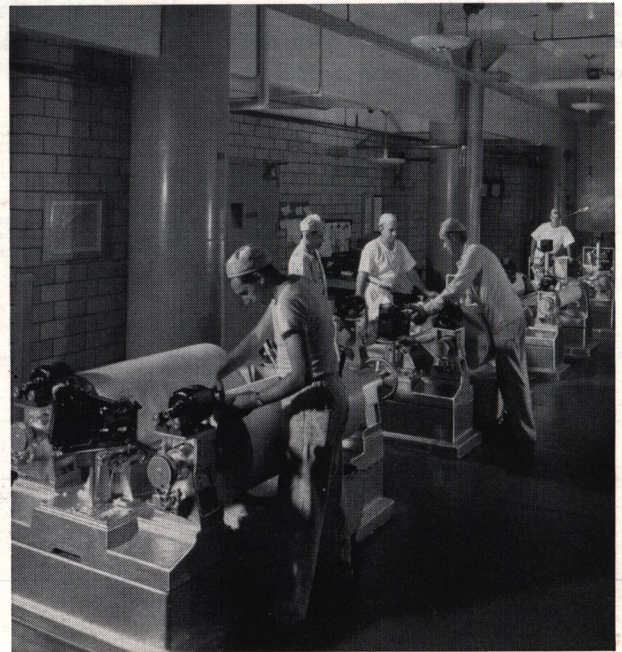
Baryta-coated paper is placed on these stock stands and drawn through a light-trap onto the sensitizing machine.
