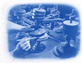
Kodak Anastigmat lens. A graphic chart shows some of the stages through which this lens goes in the course of manufacture. A big machine intrigues onlookers as it demonstrates the precise automatic grinding and polishing that help to make fine Kodak lenses available at moderate prices. Of unfailing interest also is the Newton Rings test... one of many Kodak tests on lens quality... by which lens curvatures can be checked to within a few millionths of an inch.
