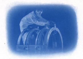
as high as a man, and weighing over a ton each, the projectors together carry 2,112 color pictures for the complete show. The whole battery is controlled by a single specially notched sound film which changes the pictures automatically, at the same time synchronizing with them special music and spoken commentary. It is only this highly complex and precise installation that makes possible the magnificent photographic effects which the visitor now sees.
