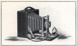
PONY Premo No. 3 has all the advantages of its two predecessors and the additional ones of rack and pinion for easy, exact focusing, long bellows draw, and double valve automatic shutter. May be loaded with films or plates and offers the ground glass focusing feature with either.
