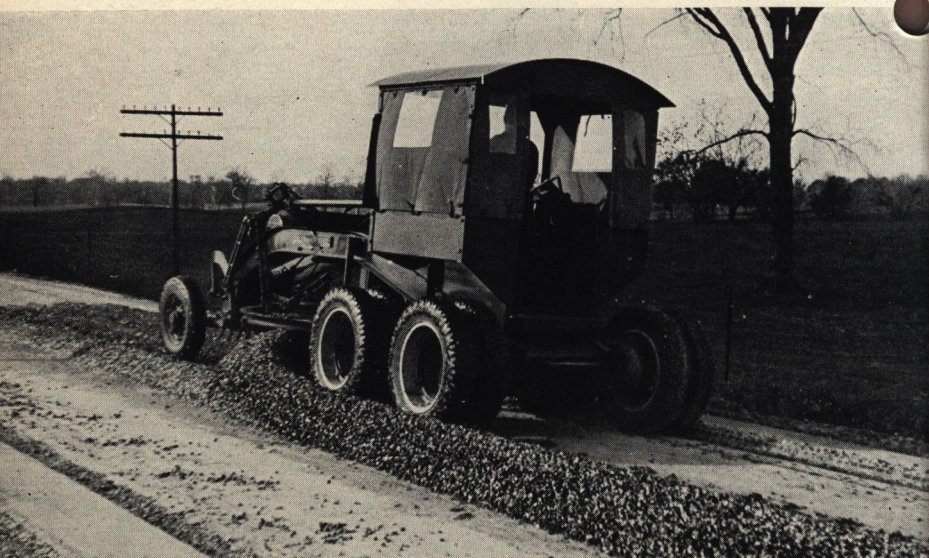
Fig. 13. LEICA photo by D. Townsend...showing Galion Patrol with double drive and dual rear tires mixing new surface material for a "retread" road surface. Lincoln Highway. Another example to show how products in actual use can be photographed for record purposes.
