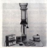
\*Kodak Colour Enlarger, Model 1 -Makes 5x7, 8x10, and 11x14 color enlargements from all sizes of photofinishing negatives up to and including 8-exposure 620. Unit includes an "integrating box" to mix and diffuse the light source to supply a high level of illumination from a 300-watt lamp, a system of sliding filters provide continuously adjustable color balance, color-control box, Galvanometer, and six glassless negative holders.
