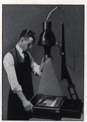
WITH this new enlarger the sharp little pictures made by miniature cameras can be enlarged from 2 1/2 to as much as 10 diameters-100 times their original negative area. The enlarger combines utmost capability and convenience. Negative capacity, up to 21/4 x 21/2 inches (or 21/4 x 31/4 inches, masking off a 21/4 x 2 1/2-inch area). Gives prints up to 16 x 24
