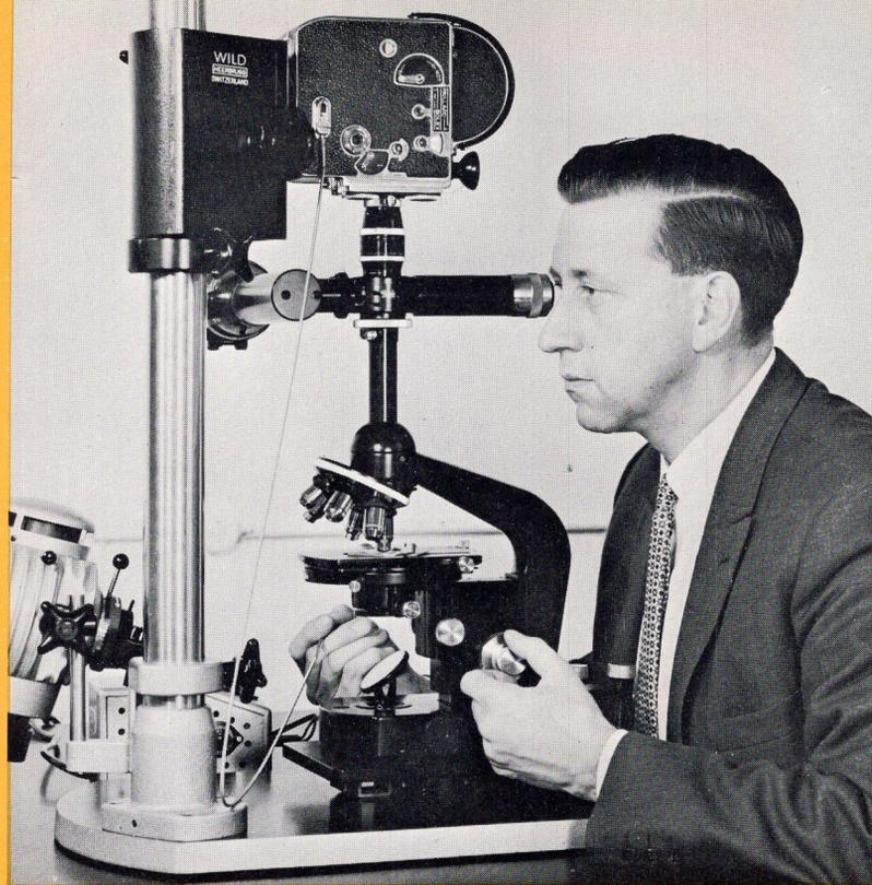
Technician engaged in Cinemotomicrography with Bolex H Camera mounted on Wild camera stand.
