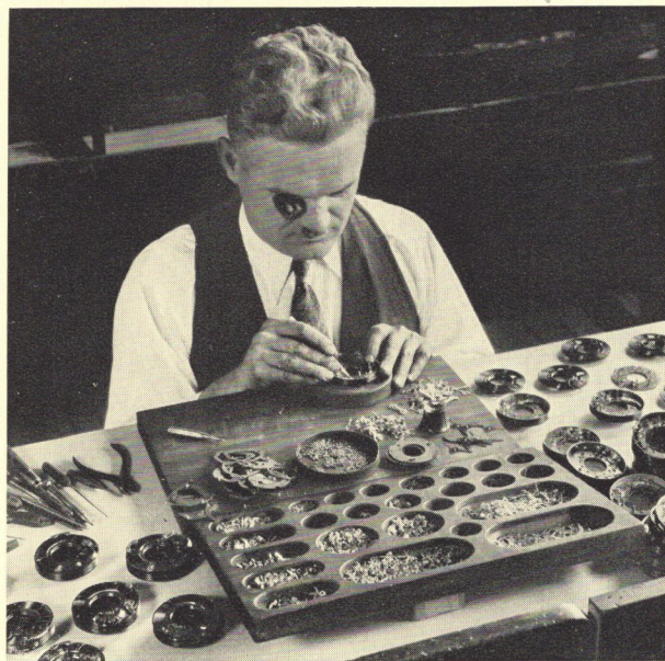
Assembling automatic shutters for Kodaks: a job for watchmakers, requiring, as it does, the delicate handling of many very small parts
