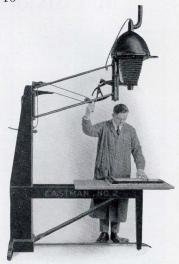
prints. This holder is fitted with movable masking arms which also hold the paper flat during the exposure. An adjustable guide may be set for white margins from  $\frac{1}{4}$  to  $2\frac{1}{2}$  inches. The printer occupies a floor space of 3 feet by 4 feet 8 inches.
